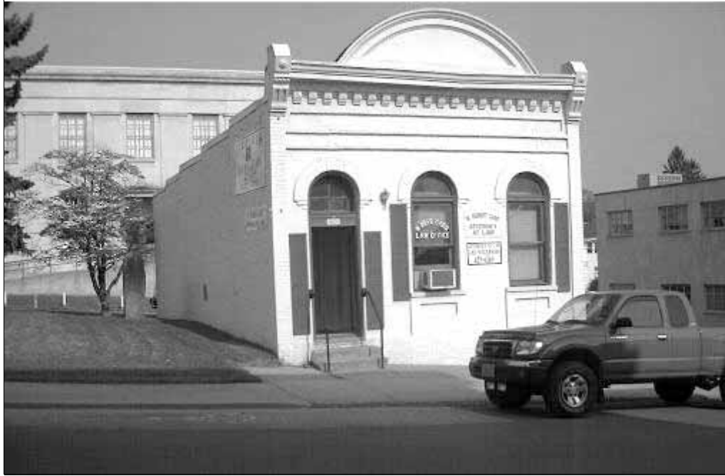
Shelton's Shoe Shop building located near Courthouse Square, Princeton, WV, where R.G. Thomas (Alva's father) had his realty business prior to 1900.
